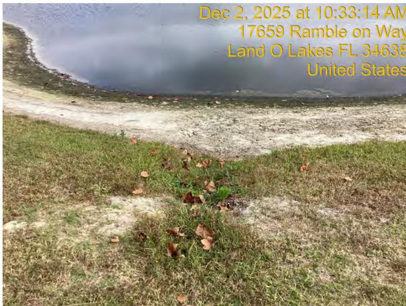
One erosion area was observed on pond 75. The location of this area is in the south west corner of the pond. The likely cause is sheet flow issues or leaking irrigation. A trench leading down to the pond is present.
