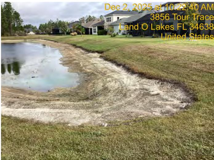
There were three main areas of erosion on pond 63. All of these areas were located along the eastern shoreline. Sheet flow issues are the most likely cause.
