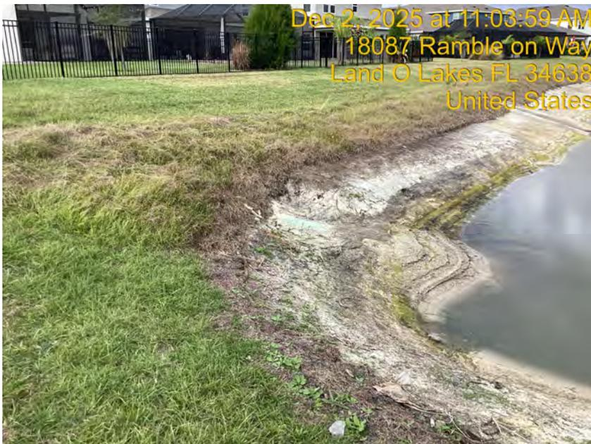
One area of erosion was observed on the recently repaired bank of pond 80. This is located in the southern corner of the pond. It has been caused by continued sheet flow issues.
