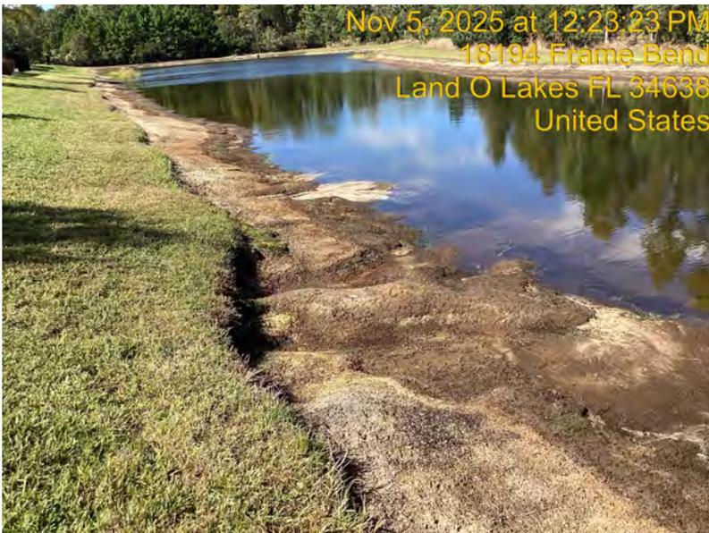
One main area of erosion was observed on pond 59, with a couple other small areas that are very minimal. The main spot of erosion on this pond was located along the eastern section of southern bank. A few minor spots to monitor were also located on the southern shoreline primarily in between houses.
