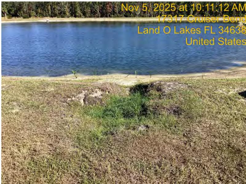
One area of erosion was observed on pond 52. This area was located on the north eastern shoreline. This spot was caused by sheet flow issues.
