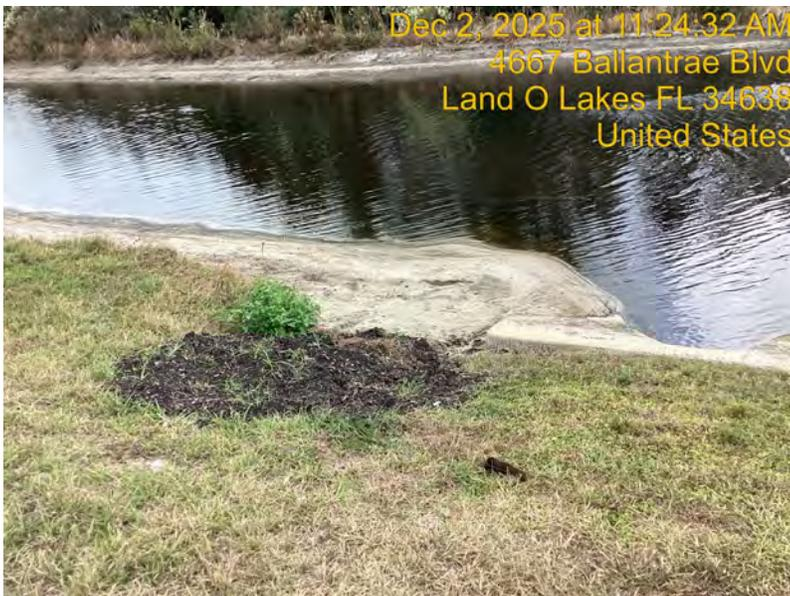
One area of erosion was observed on pond 60. This area was likely caused by sheet flow issues. This area was filled in with mulch, most likely by one of the homeowners.
