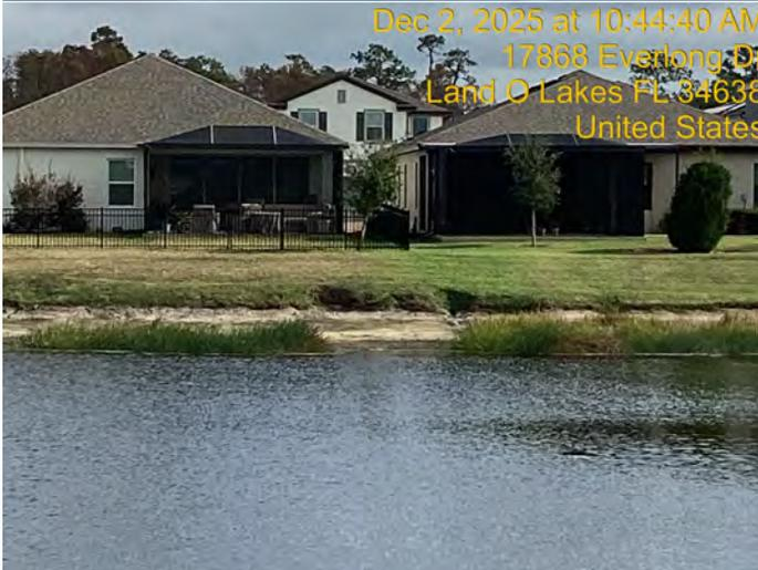
Significant erosion areas were observed on pond 79. Three main areas are pictured. They are located on the northern and eastern shorelines. These were caused by sheet flow issues. Due to extended periods of exposed sediment with no structural support, rain events have further progressed the erosion areas.
