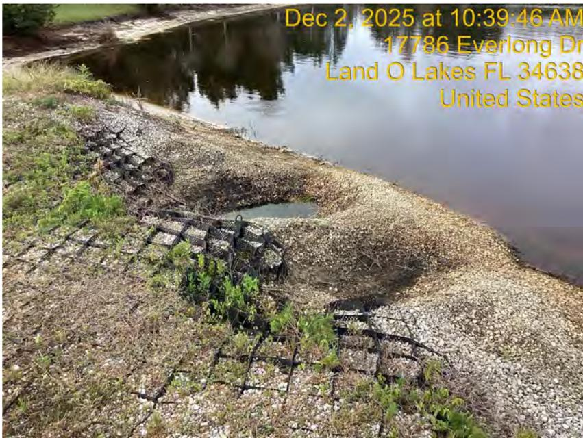
The rock area on pond 77 should be filled in more. In addition to that, sheet flow issues has caused to holes to form on the shoreline in this area. This is located along the eastern shoreline.
