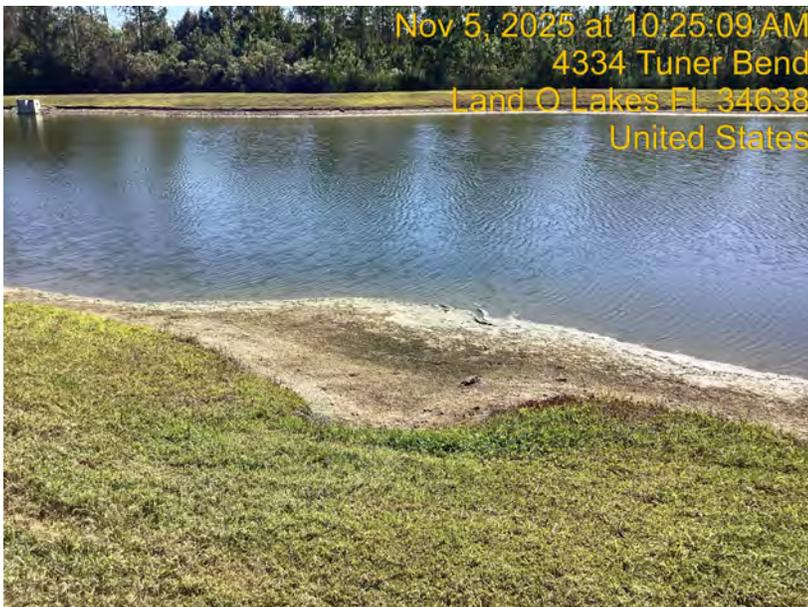
One erosion area was observed on pond 50. This area of erosion was located along the north western bank. The cause for this erosion is likely due to sheet flow issues.
