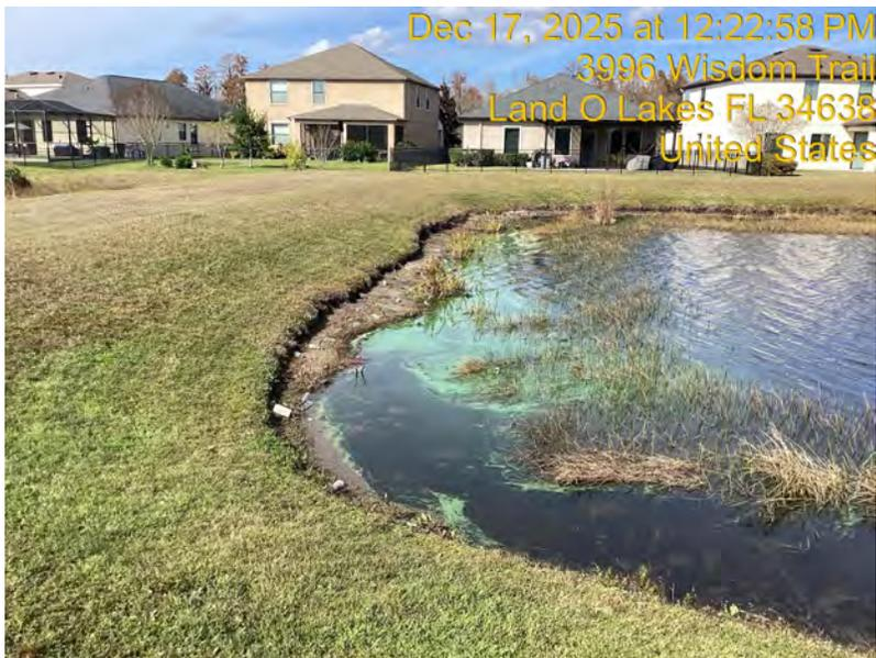
Pond 8 has one area where erosion was observed. The south western bank has minor wind wave action erosion along the shoreline.
