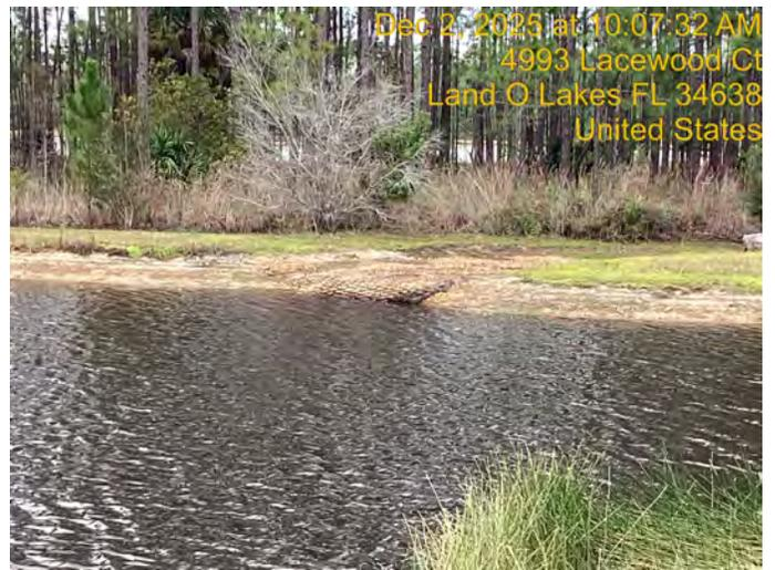
One erosion issue area was observed on pond 67. The erosion in this area was likely caused by sheet flow issues. The rock area on this pond should also be filled in more.
