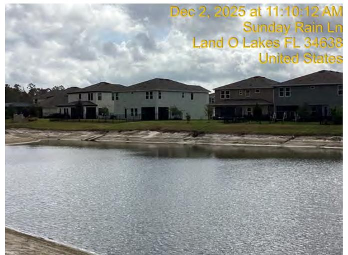
Several erosion areas were observed on pond 81. Sheet flow issues and prolonged low water levels have exacerbated these issues. The southern shoreline is the primary location for the majority of the erosion areas.
