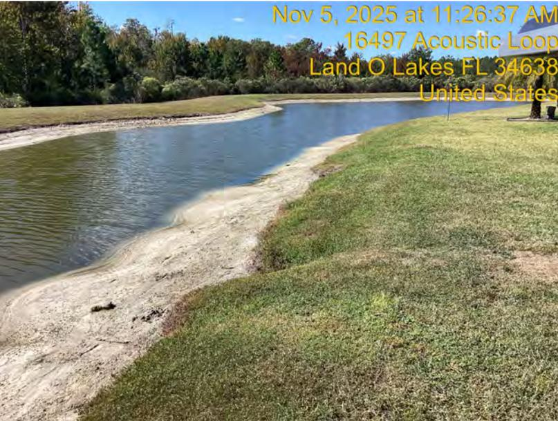
Two areas where observed with erosion on pond 38. Both locations appear to be caused from sheet flow issues from between houses.
