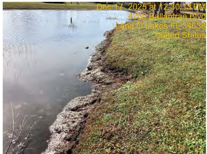
Pond 6 has two areas with erosion observed. The area pictured on the left looks to be caused by the flow of out of the wetland area and into the pond. The area pictured in the right image was caused by sheet flow issues. Both of these areas do not appear to have any changes recently, but could potentially worsen over time.
