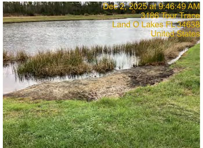
One area of erosion was observed on pond 71. This area was located in the north west corner of the pond. Sheet flow issues have caused erosion and a trench going down to the pond.
