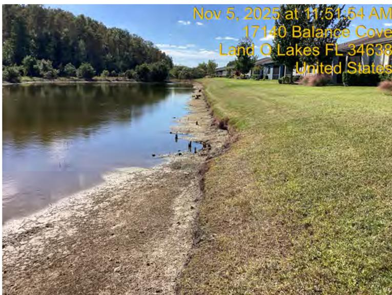
Pond 26 has one area of erosion that was observed. This area is a roughly 10ft length, where the shoreline has receded back 1-2ft. This area is located near the north western corner of the pond.
