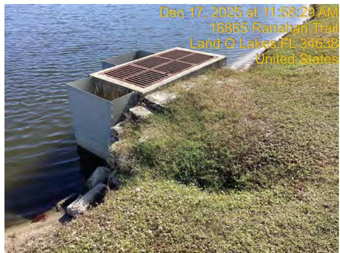
Pond 25 has two main areas where erosion was observed. In the left picture, a section of the north western shoreline can be seen with several erosion pockets that have been caused by sheet flow issues. In the left picture another sheet flow issue has lead to erosion near the outflow structure and is a hole. The area near the outflow structure should be addressed soon.
